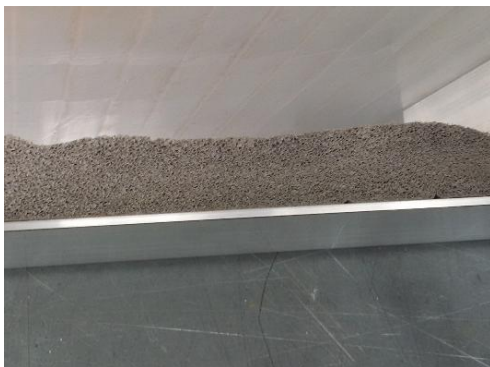
Figure 35 Expanding sealant tape right after application
