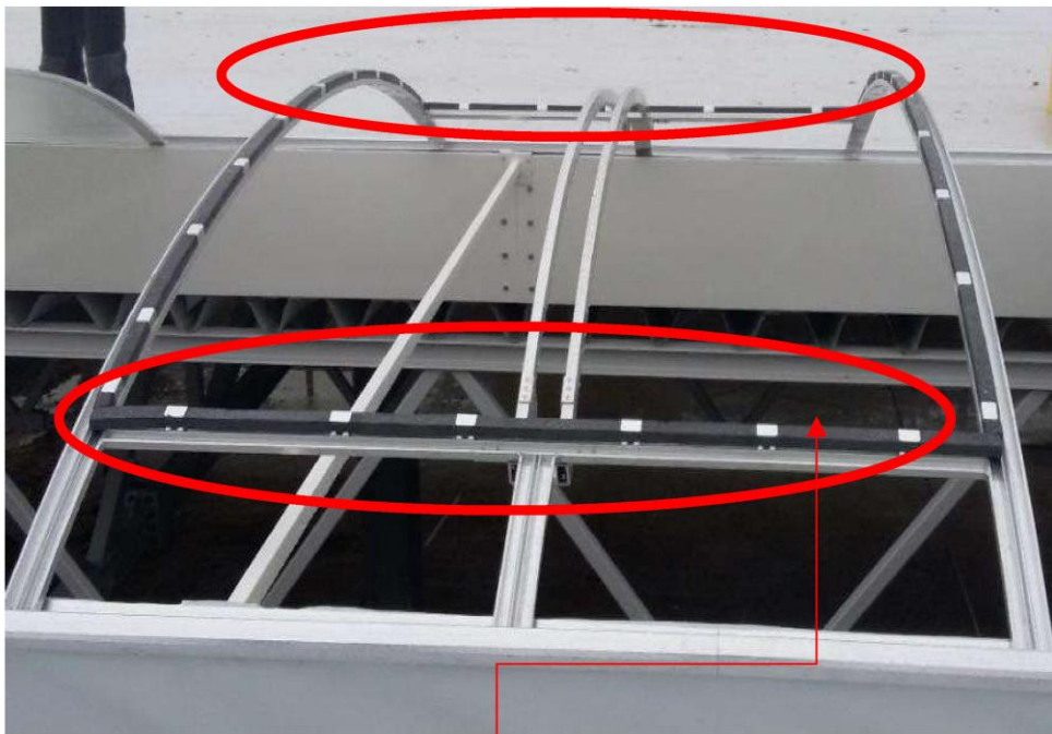
Figure 48 Layout of brackets on the vent support frame
